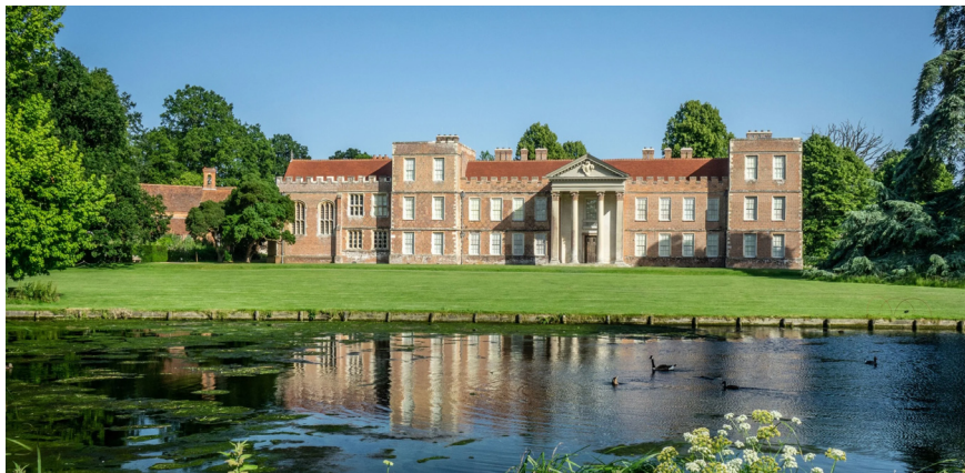
The Vyne, north façade
